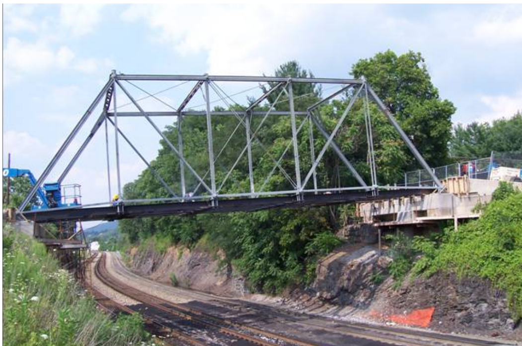
Figure 5.1 Hawthorne Street Bridge, Covington, Virginia
